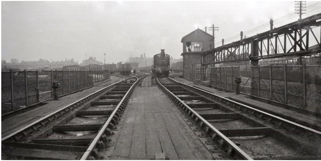
Looking over the Swing Bridge towards Rewley Road Station and Goods Yard, behind the locomotive, with fixed gantry leading to the signal box. The Shipley Coal Sidings, oil depot & Axtell & Perry stone yard are on the left of locomotive. c 1930
