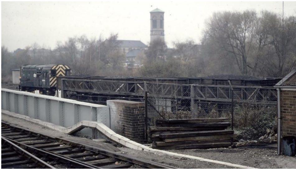
Locomotive propelling loaded coal wagons into Shipley Sidings. The fixed span carrying the signal wires and rodding can be seen at the side of the wagons. The fixed span was removed in 1981
