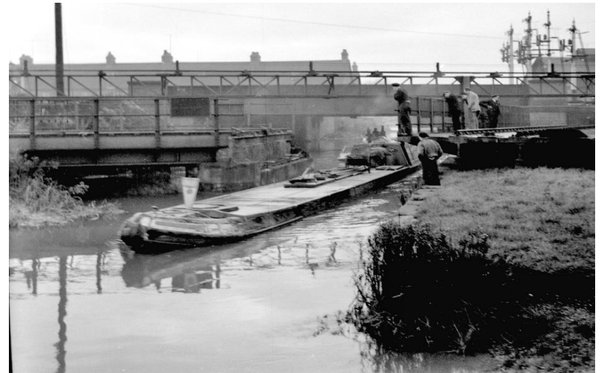
Barge passing through whilst the four bridge operators remain on the Swing Bridge to wind it back to its fixed position as there was no safe way for the operators to leave the structure to return to the Rewley Road Station side. 1956
