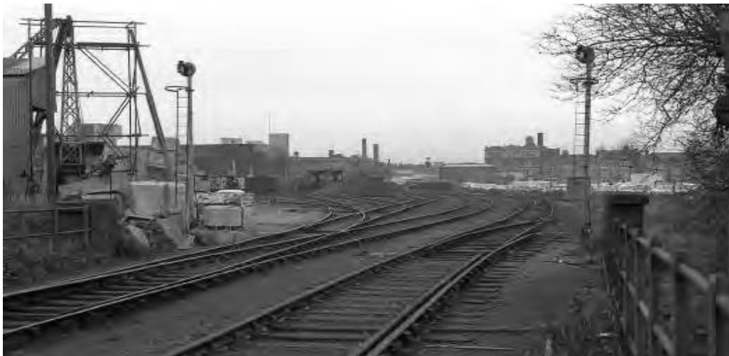
Looking towards the Station and the Jam Factory in the distance, with the stone mason's crane the Shipley Sidings on the left. The two raised disc signals were controlled from the ground frame on the Bletchley side of the Swing Bridge after the signal box closed in 1956 and was demolished in 1965
