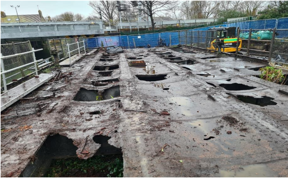
Restoration work in progress – Removal of the 1890's deck plates in 2021
